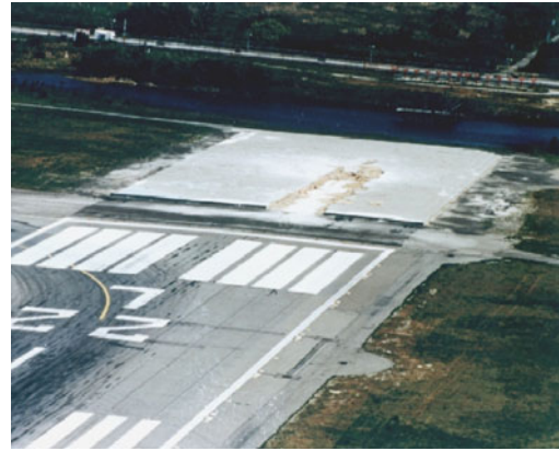
Figure 5 - Photos of EMAS off Runway 22L at JFK taken the day after the safe arrestment of a SAAB-340 overrun in June 1999 (note the surface area removed to extract the aircraft)
