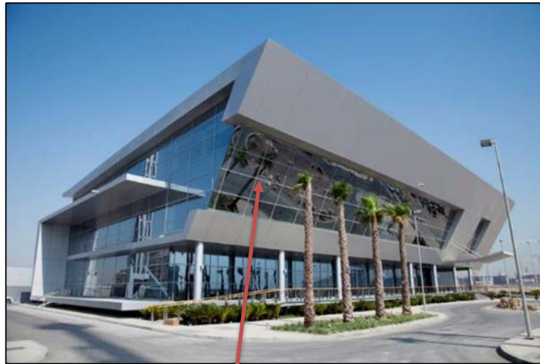
MID FPP Manager Office
