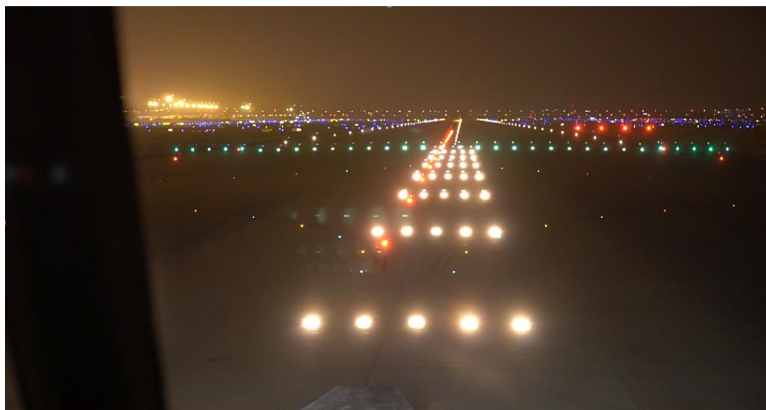
Figure 2 Testing Take-off Hold Lights at Shanghai Hongqiao Airport
