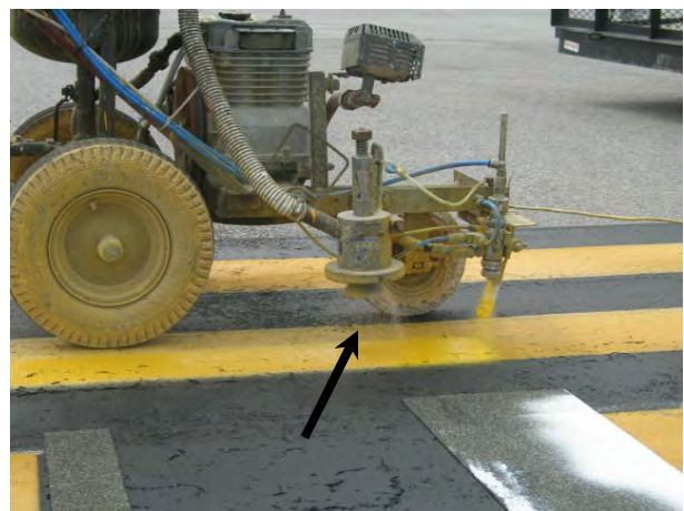
FIGURE 6-41. GLASS BEAD DISPENSER ON AN ATOMIZED HAND MACHINE.
