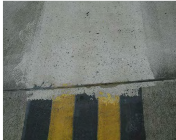
FIGURE 5-9. ON CONCRETE, CARE WAS EXERCISED TO AVOID DAMAGE.
