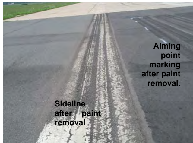
FIGURE 5-27. BEFORE PAINT REMOVAL. FIGURE 5-28. AFTER PAINT REMOVAL.
