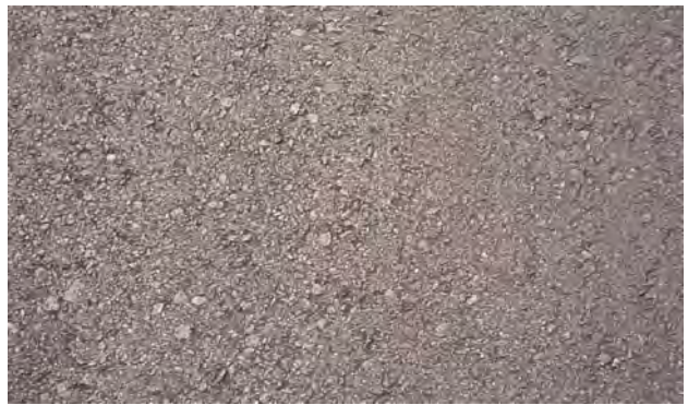
FIGURE 4-10. AFTER RUBBER REMOVAL.
