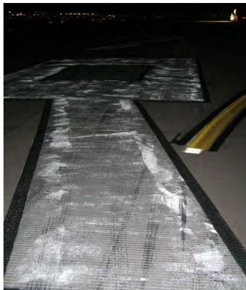
FIGURE 6-49. VISIBILITY OF THE “R” IS POOR AT NIGHT.
