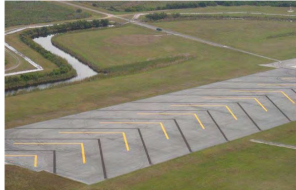
What appear to be black chevrons were old ones, removed since they conflicted with the new layout. Ultraviolet light will soon fade the unexposed, black asphalt to gray.
