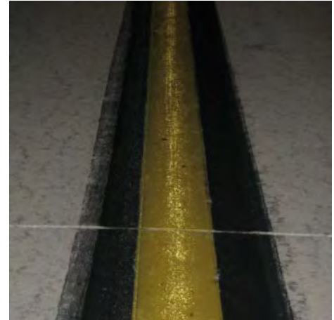
FIGURE 3-9. NON-FUNCTIONAL MARKING DUE TO POOR REFLECTIVITY.
