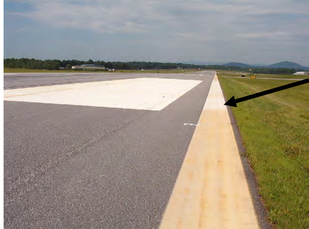
FIGURE 4-25. GROOVED SURFACE MAKES STAIN LESS NOTICEABLE.
