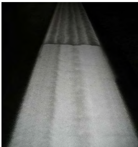
FIGURE 6-31. PRESSURIZED BEAD APPLICATION IN FOREGROUND, GRAVITY-DROP IN BACKGROUND.
