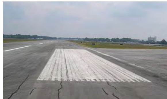
FIGURE 4-17. AFTER WATERBLASTING, BUT BEFORE PAINTING.
