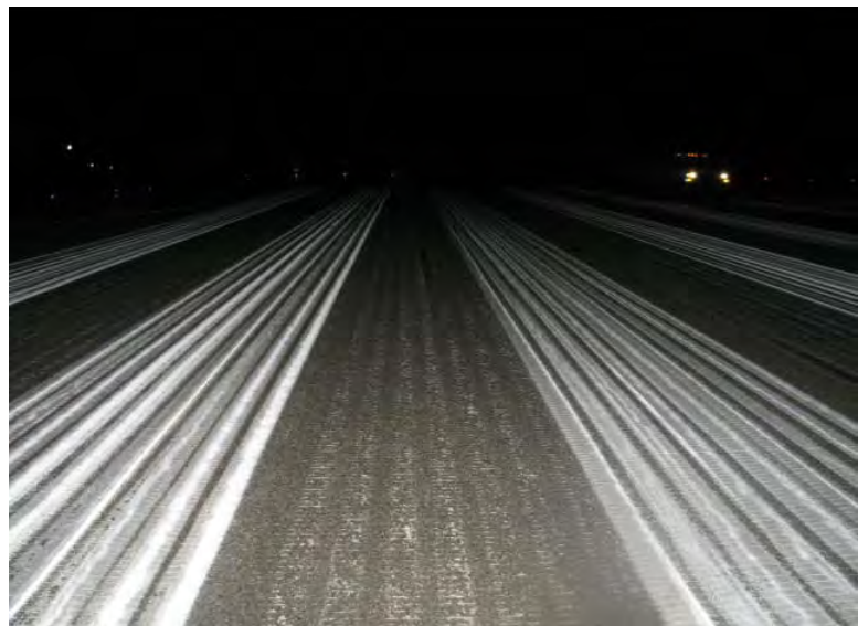
FIGURE 6-17. STRIATED MARKINGS ARE NOT AS VISIBLE AS SOLID MARKINGS; AND WHEN BEADS ARE POORLY APPLIED, THEY ARE DIFFICULT TO SEE DURING LOW-VISIBILITY.
