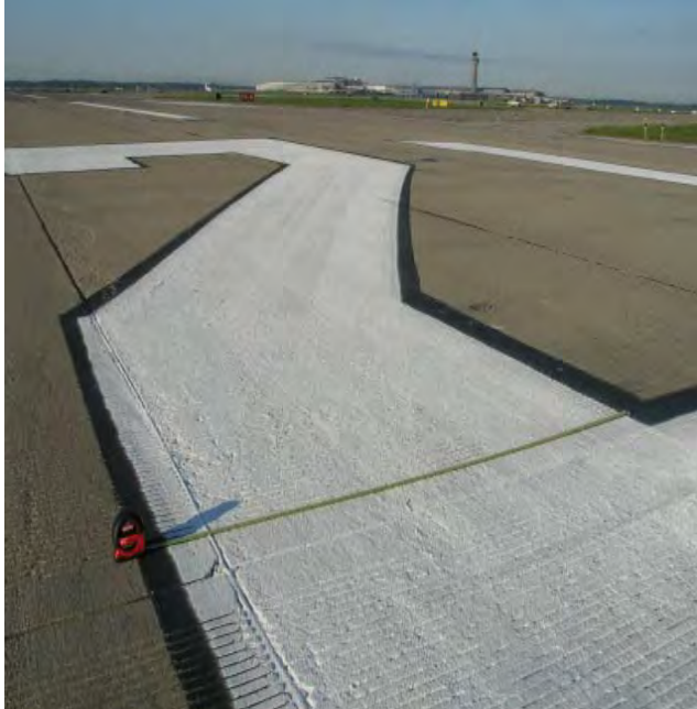
FIGURE 2-2. MEASURE EXISTING MARKINGS TO DETERMINE COMPLIANCE WITH AC 150-5340-1.
