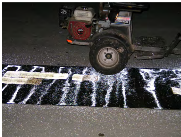
FIGURE 6-58 TEST LINES ON TAR PAPER.
