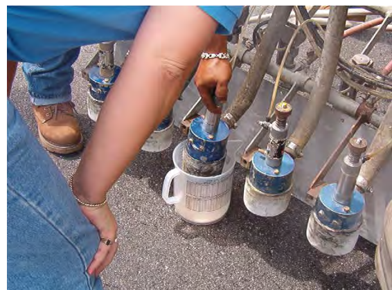
FIGURE 6-60. CALIBRATION OF GLASS BEAD GUNS.
