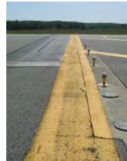
What appear to be black chevrons were old ones, removed since they conflicted with the new layout. Ultraviolet light will soon fade the unexposed, black asphalt to gray.
