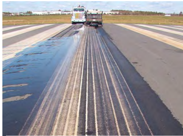
FIGURE 5-18. HIGH-PRESSURE WATERBLASTING IS EFFECTIVE FOR CLEANING LOOSE AND POORLY BONDED PAINT (SURFACE PREPARATION).
