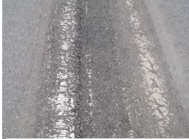
FIGURE 5-30. REMOVAL OF MULTIPLE LAYERS ON DETERIORATED ASPHALT.
