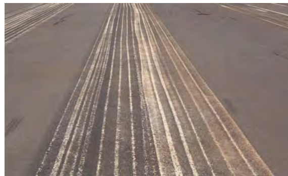
FIGURE 4-2. AFTER CLEANING LOOSE AND POORLY BONDED PAINT BY WATERBLASTING.
