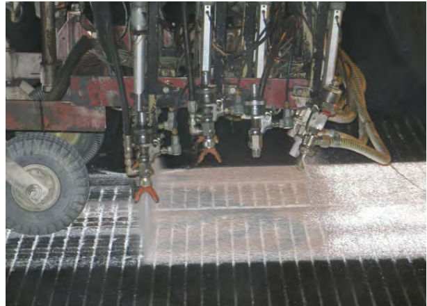
FIGURE 6-21. AIRLESS PAINT GUNS AND BEAD GUNS APPLYING MATERIAL TO PAVEMENT.
