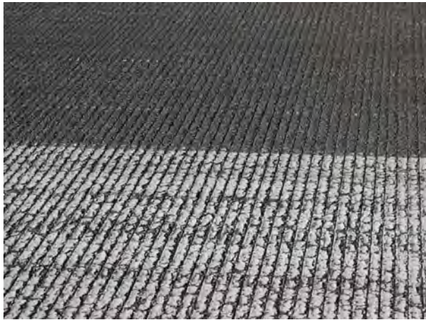
FIGURE 5-22. MARKING BEFORE (BOTTOM) AND AFTER (TOP) REMOVAL.
