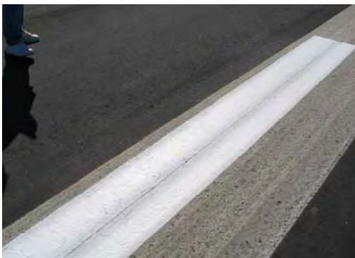
FIGURE 6-46. UNEVEN MATERIAL DISTRIBUTION, LIGHT ON THE EDGES OF EACH PAINT GUN.
