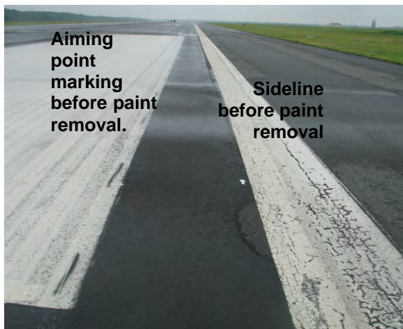
FIGURE 5-27. BEFORE PAINT REMOVAL. FIGURE 5-28. AFTER PAINT REMOVAL.
