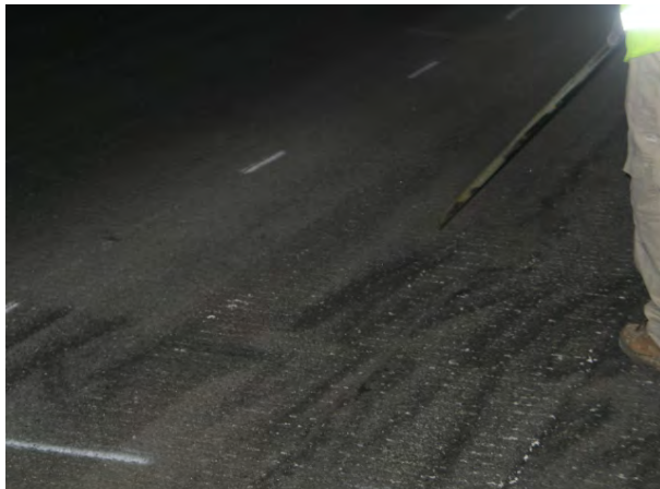
FIGURE 4-37. COMPRESSED AIR REMOVES FINE RESIDUE AFTER PAINT REMOVAL OPERATION.
