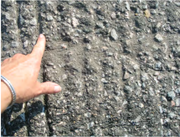
FIGURE 5-12. AFTER REMOVAL OF THE MARKINGS ON GROOVED PAVEMENT WITH SHOTBLASTING.
