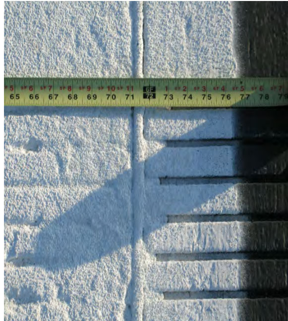
FIGURE 2-3. MARKING DIMENSION IS OUT OF TOLERANCE.
