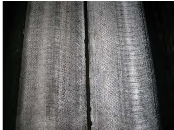
FIGURE 4-40. HEAVY RUBBER DEPOSITS WERE REMOVED FROM THIS CENTERLINE MARKING WITH ULTRA HIGH-PRESSURE WATERBLASTING.
