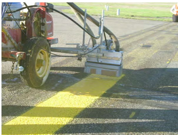
FIGURE 6-40. GLASS BEAD DISPENSER HAS BEEN MODIFIED WITH A CARDBOARD WINDSCREEN.
