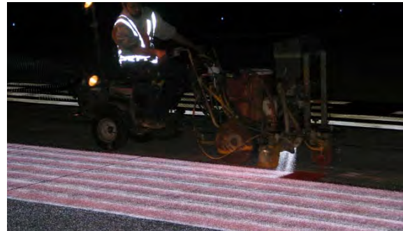
FIGURE 6-39. AN AIRLESS MACHINE WITH A MOTORIZED “SULKY” APPLIES MARKING WITH AUTOMATIC GLASS BEAD GUNS.
