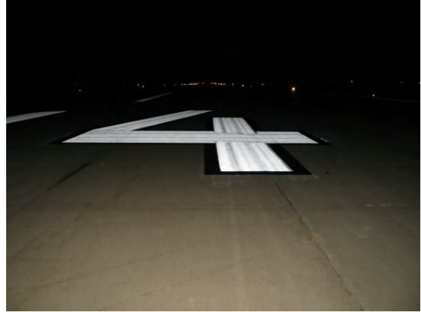
FIGURE 6-52. NIGHTTIME VISIBILITY OF FIGURE 6-51 IS EXCELLENT.
