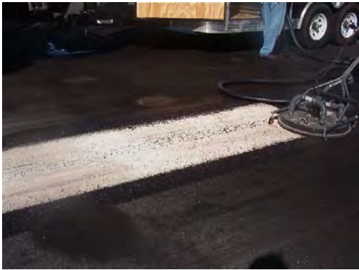
FIGURE 4-34. THE PROCESS USED TO REMOVE OIL STAIN.
