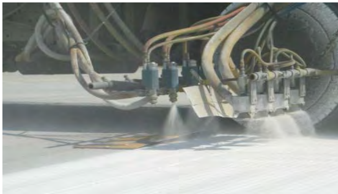
FIGURE 6-28. FOUR PNEUMATIC (ATOMIZED) PAINT GUNS APPLYING A 3-FOOT WIDE PATTERN.
