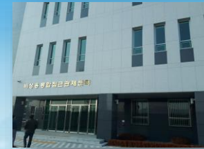
KASS Operation Center #1 (Chungju)
