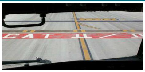
ENHANCED ILS DESIGNATOR MARKING AT PATTERN B HOLDING POINT DESIGNATOR PLACED ACROSS THE TAXIWAY AT 45M INTERVALS IF THE TAXIWAY EXCEEDS 60M IN WIDTH TO INDICATE CAT II OR CAT III HOLD POINT
