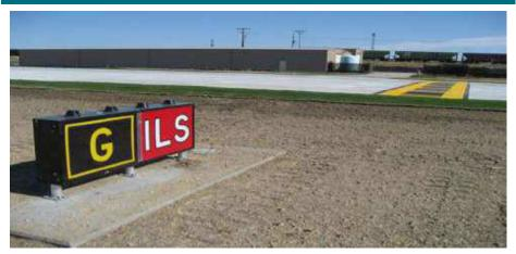
CRITICAL ILS BOUNDARY MANDATORY SIGN AT PATTERN B HOLDING POINT VARIATION RECOMMENDED BY FAA WHERE MANDATORY HOLDING POINT FOR ILS HOLD IS NOT IDENTIFIED BY ADDITIONAL RUNWAY DESIGNATOR
