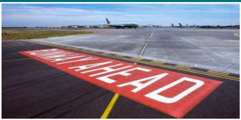
ENHANCED MARKING WARNING OF RUNWAY (UNABBREVIATED) AHEAD TRIALLED BY UKCAA AND BAA AT LONDON HEATHROW (LHR) BUT WITH NO ENHANCED CENTRELINE TO STRENGTHEN THE RUNWAY AHEAD WARNING
