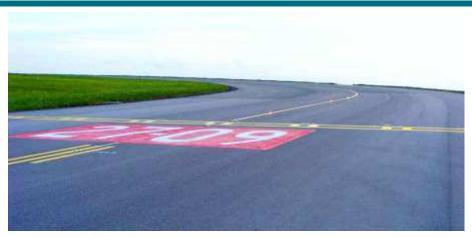
ENHANCED RUNWAY DESIGNATOR MARKING AT PATTERN B HOLDING POINT DESIGNATOR PLACED CENTRALLY ACROSS THE TAXIWAY CENTRELINE INDICATING UP TO CODE D IMMEDIATELY BEFORE THE CAT II HOLDING POINT
