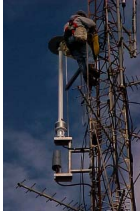
Figure 5 -- Mode S 1090ES ADS-B and Multilateration Antennas Installed On Existing Communication Tower On Representative Oil Platform
